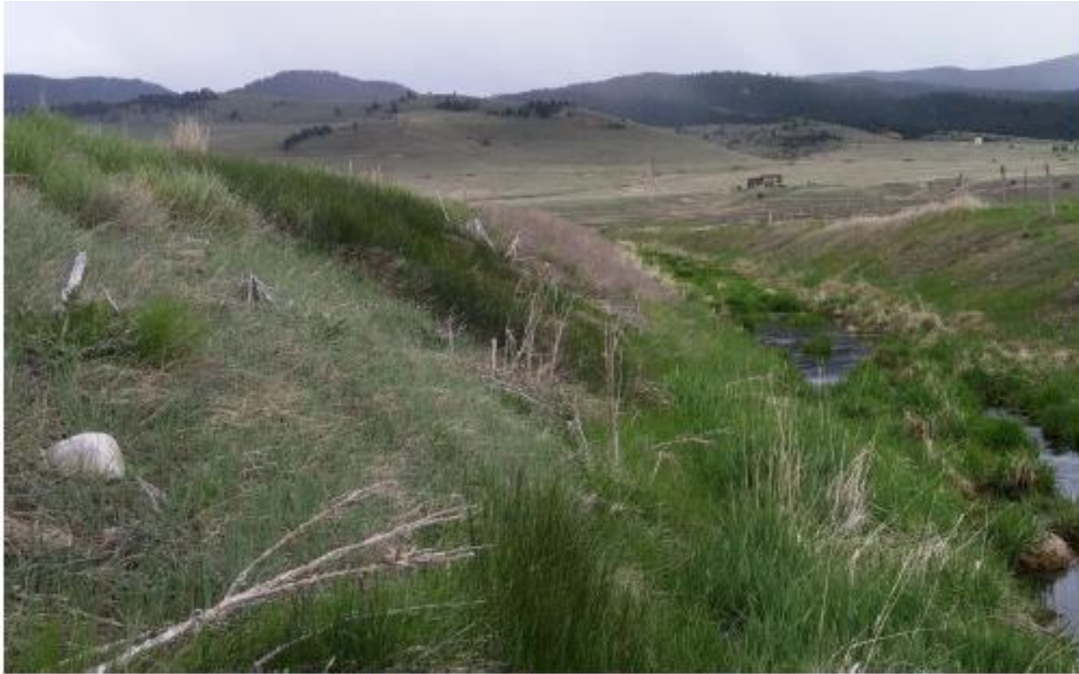
Figure 3. Outside of Cell 2 at Southwest Corner
